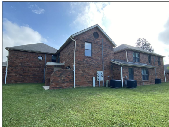
3 A1.2 NTS EXTERIOR PHOTOGRAPH
