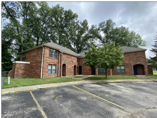
3 EXTERIOR PHOTOGRAPH A1.4 NTS
