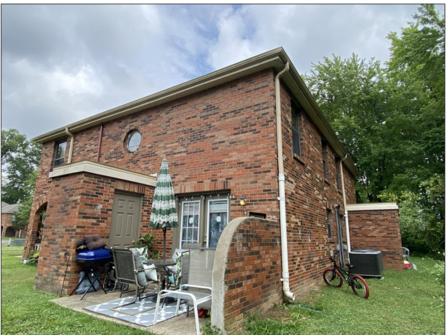
2 EXTERIOR PHOTOGRAPH A1.3 NTS
