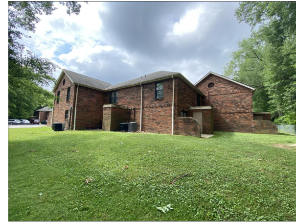
6 EXTERIOR PHOTOGRAPH A1.4 NTS
