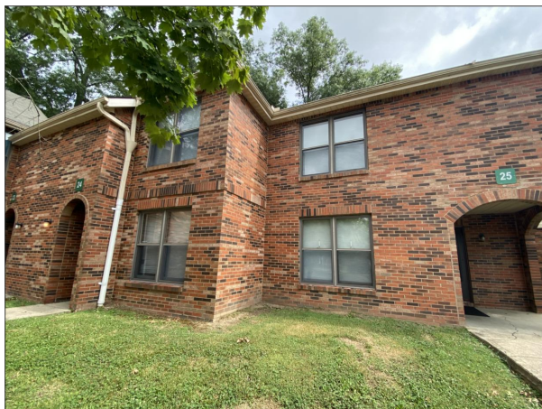
2 EXTERIOR PHOTOGRAPH A1.4 NTS
