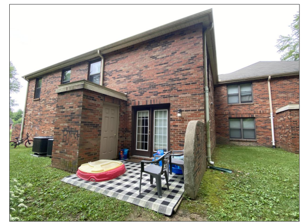
6 EXTERIOR PHOTOGRAPH A1.3 NTS
