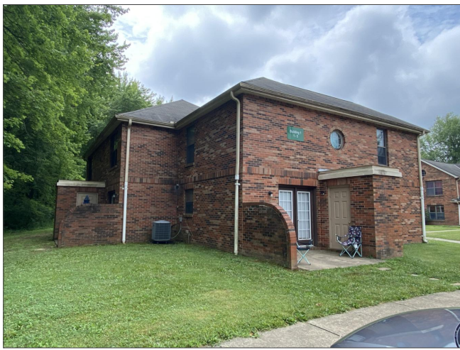
4 EXTERIOR PHOTOGRAPH A1.3 NTS
