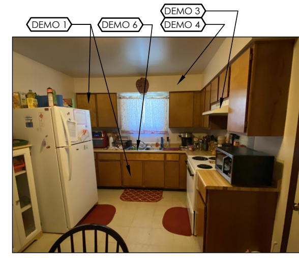
EXISTING KITCHEN PHOTO (NOT TO SCALE) 155 N SIXTH ST, BATAVIA, OHIO 45103
