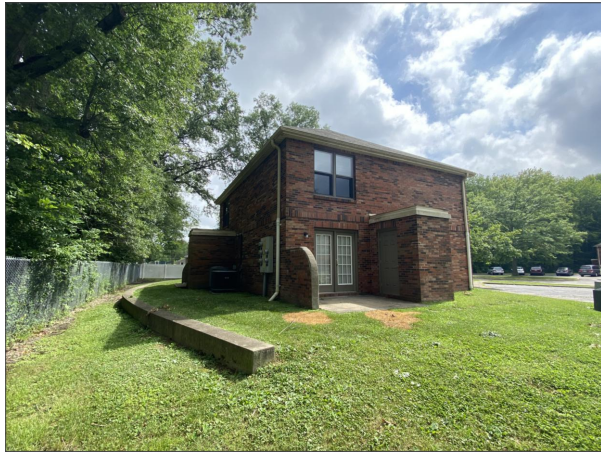
4 EXTERIOR PHOTOGRAPH A1.4 NTS
