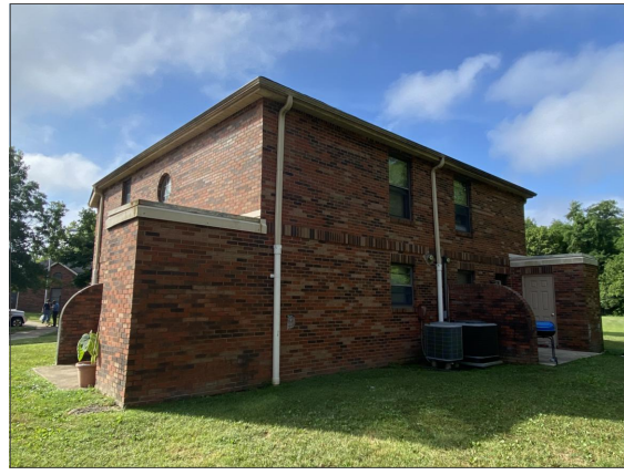
5 A1.2 NTS EXTERIOR PHOTOGRAPH
