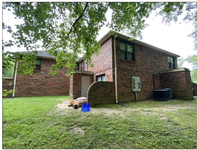
5 EXTERIOR PHOTOGRAPH A1.3 NTS
