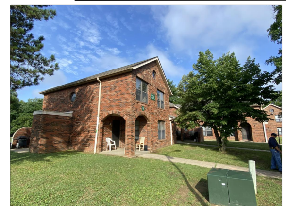
7 A1.2 NTS EXTERIOR PHOTOGRAPH
