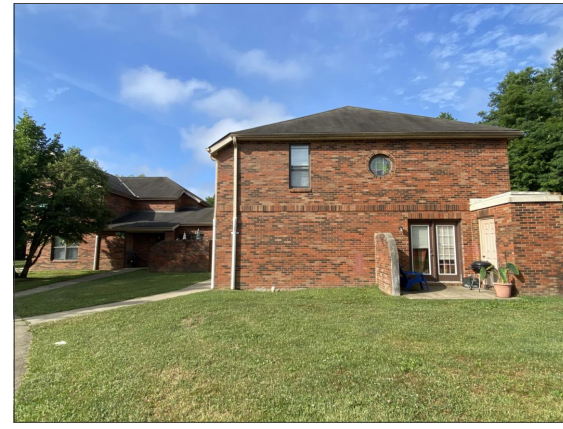
6 A1.2 NTS EXTERIOR PHOTOGRAPH
