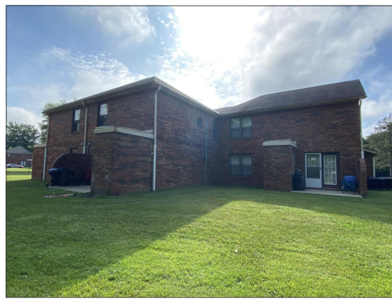
4 A1.2 NTS EXTERIOR PHOTOGRAPH
