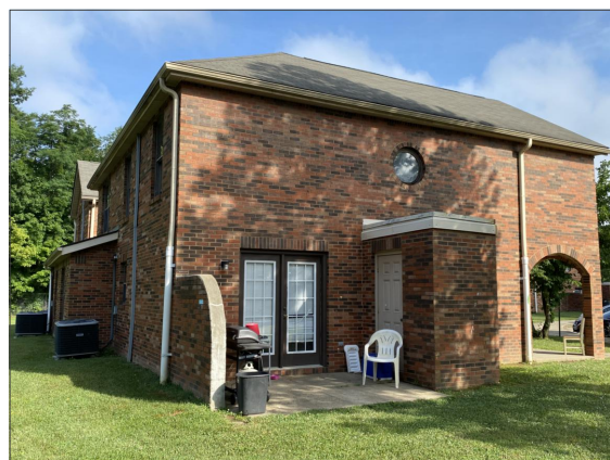
2 A1.2 NTS EXTERIOR PHOTOGRAPH
