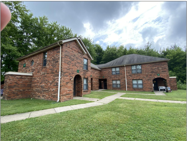
3 EXTERIOR PHOTOGRAPH A1.3 NTS
